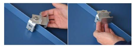
5. After the top mounted bolt on the RCB-2 Swivel Bracket is torqued to the desired setting, center the SnoCleat in the bracket and install by securing with the (2) supplied Tek screws.
