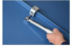
3. Install the RCB-2 Swivel Bracket with top mounted bolt and washer on top of the SnoCleat Roof Clamp and torque to 100 inch/lbs. The RCB-2 Swivel Bracket can be torqued to a lower setting to help protect the seams in the event of a heavy snow impact. The RCB-2 Swivel Bracket should always be placed downslope to support the SnoCleat.
